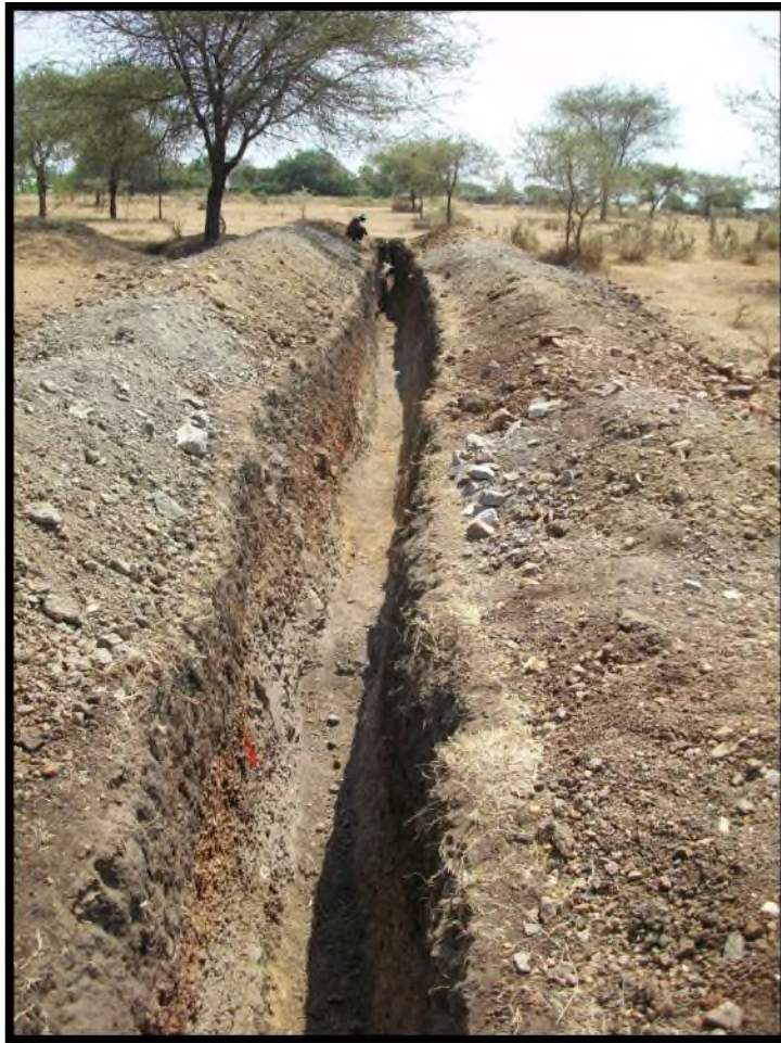
Photograph 4. North Trending Excavated to Granitic Bedrock in the Kanunga 1 Gold Prospect; Two Meter Channel Samples Taken at the Base of the West Wall (photograph from King and Barber (2011)).
